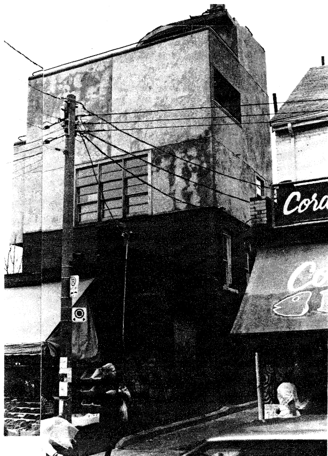
Fig. 3. Kensington Tower, Baldwin St., Toronto
