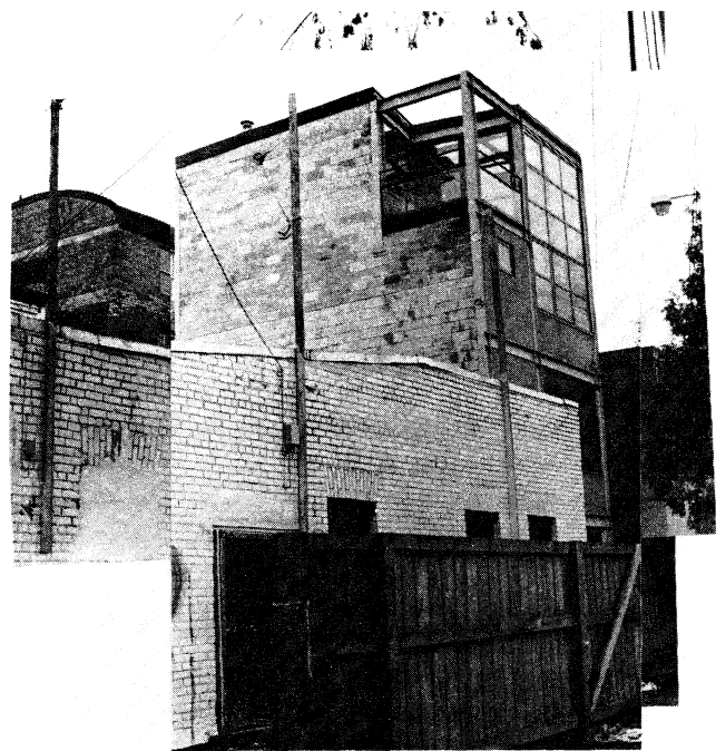
Fig. 4. Tower addition to 1024 Queen St. west, Toronto, view from lane.
